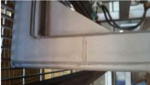
Excellent surface cleaning at weld seams.
