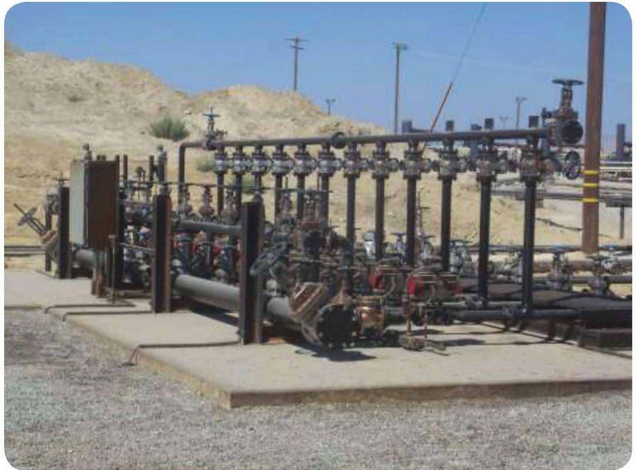
FIGURE 1 Steam injection platform.
