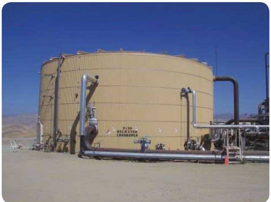
FIGURE 2 A 10,000-bbl produced water tank.
